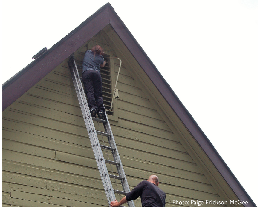
POSSIBLE ENTRY POINT FOR BATS: GABLE ENDS.
