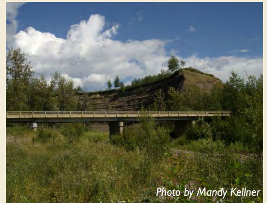
A concrete bridge in B.C. used as a roost site by Myotis bats.
