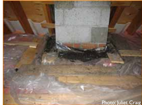
MODIFICATIONS FOR BAT ROOST SITES: PLASTIC SHEETING IN ATTIC TO FACILITATE GUANO REMOVAL AND REDUCE SMELL.
