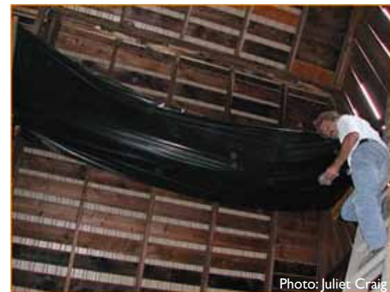
MODIFICATIONS FOR BAT ROOST SITES: TARP HUNG TO PREVENT GUANO FROM FALLING ON HAY.
